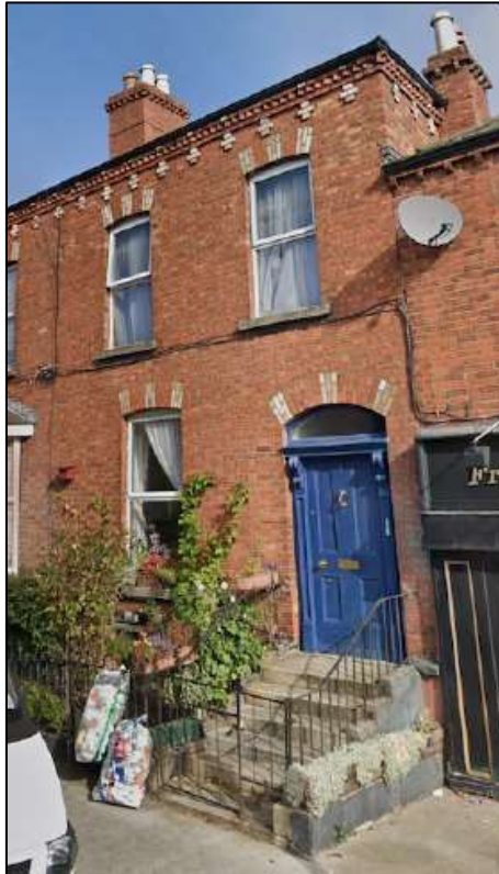
Above: 2 St Vincent's Street North. Source: Google Street View.
