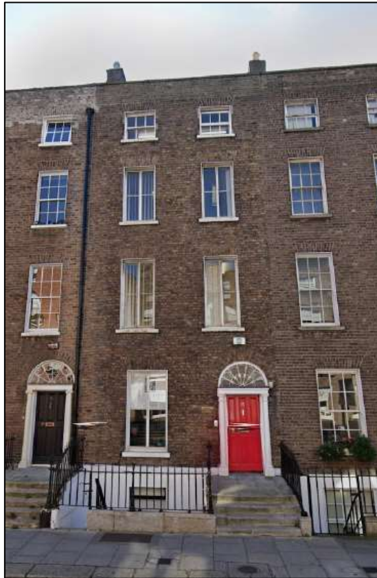
Above: 13 Pembroke Street Upper. Source: Google Street View.
