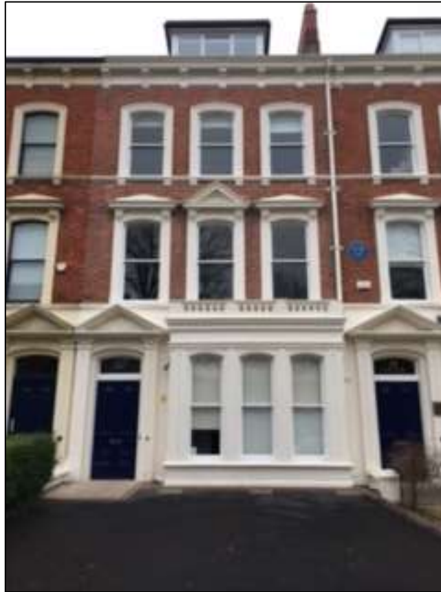
Above: 24 College Gardens. Source: Google Street View.
