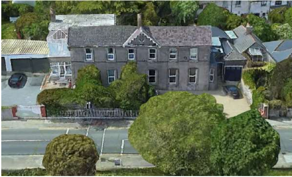
Above: 169 Strand Road. Source: Google Street View.
